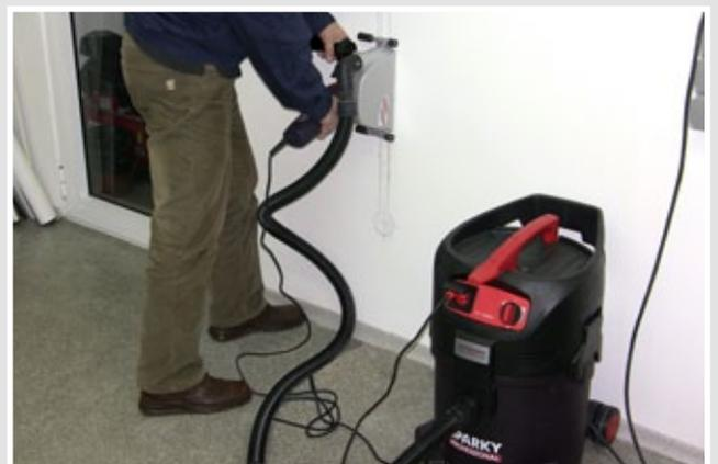
**Comes complete with:** 2 diamond discs, Disc guard with rollers, Dust extraction port, Anti-vibration side handle, Support washer, Lock nut, 6 thrust washers, Lock nut spanner
